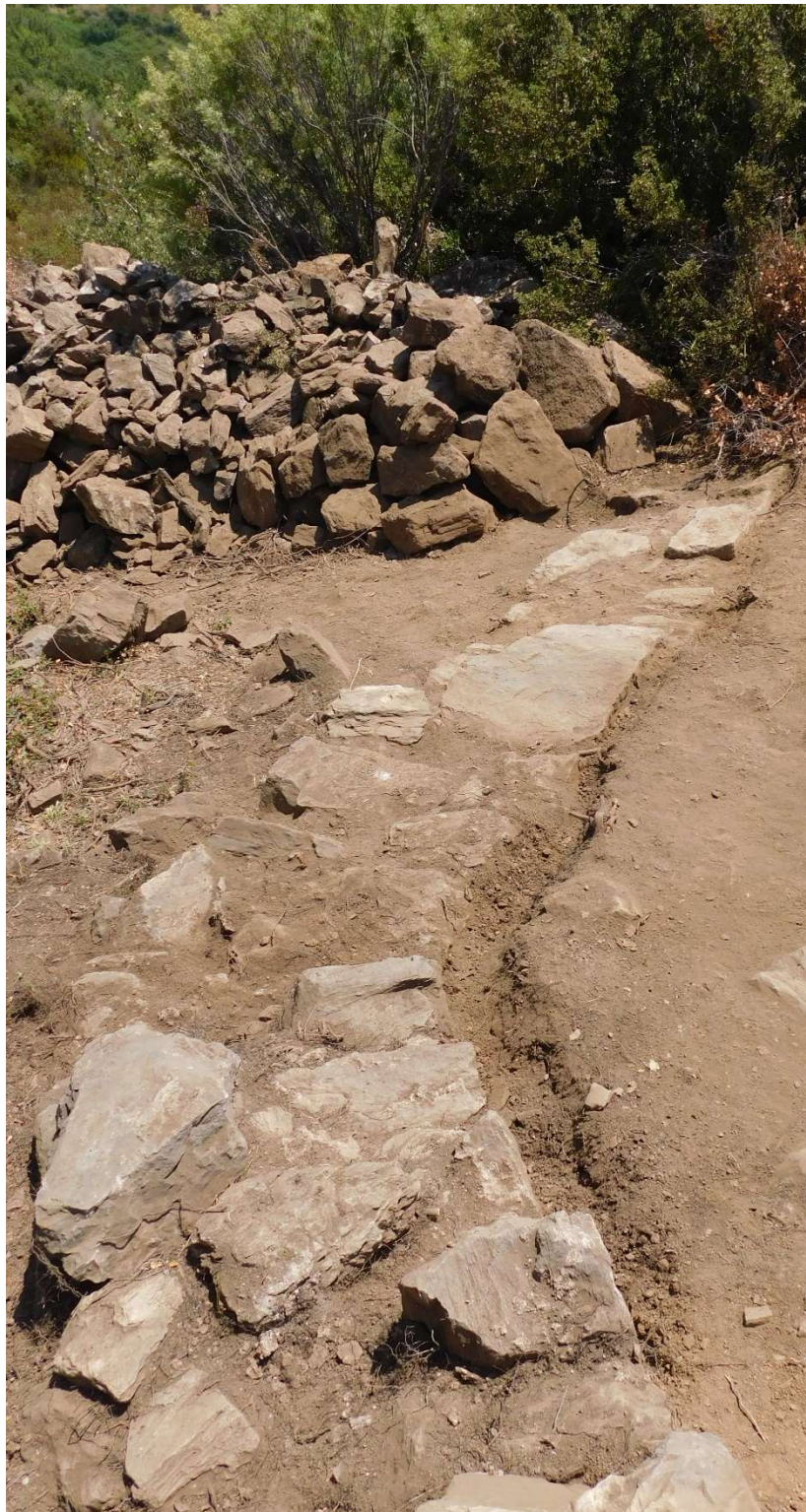
Figure 4: Wall to the Adjacent Room
