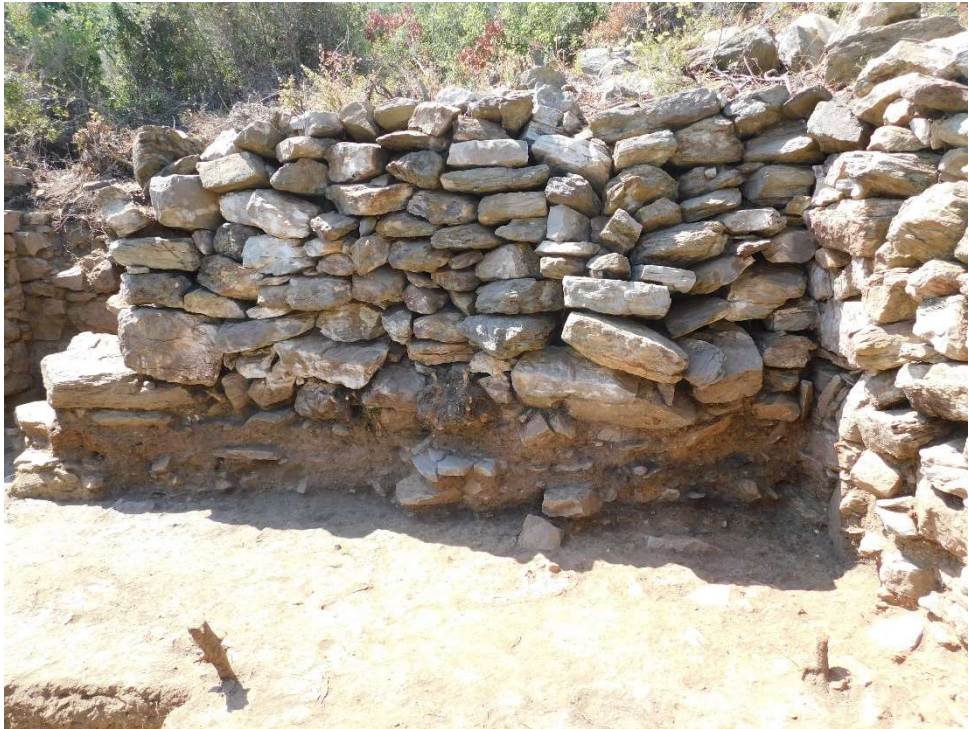
Figure 10: Poorly Built Southeast Wall
