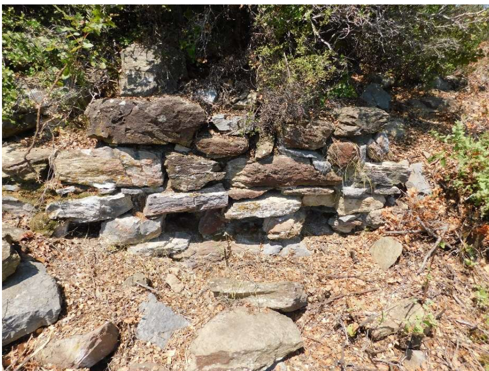
Figure 1: Wall with Beam Holes
